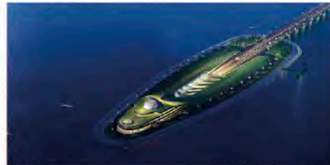
Man-made Island of Hong Kong-Zhuhai-Macao Bridge, 2017
